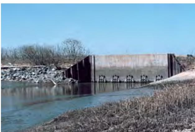
**Figure 6.5** The tide gate at the mouth of Army Creek on the Delaware side of the Delaware River. The tide gate drains flood and rain water out of the creek to prevent flooding. The five circular mechanisms on the gate open and close to control water flow [Photo source: courtesy NOAA Photo Library].
