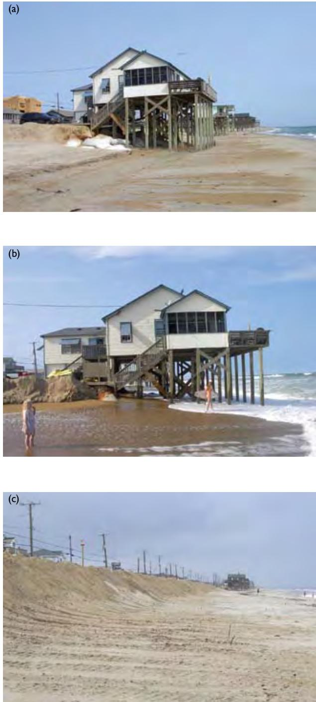
**Figure 12.6** Retreat. (a) June 2002. Houses along the shore in Kitty Hawk, North Carolina. Geotextile sand bags protect the septic tank buried in the dunes. (b) October 2002. (c) June 2003 [Photo source: ©James G. Titus, used with permission].
